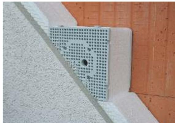
**Assembling installation box into thermal insulation MDZ**
